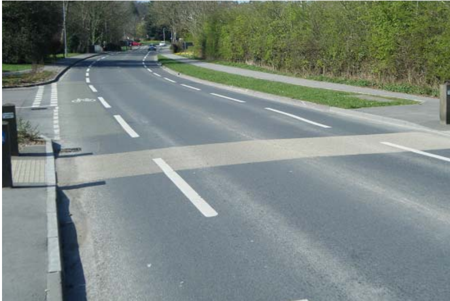
Picture 16.5 Removal of centre line with cycle lanes, Laverstock
